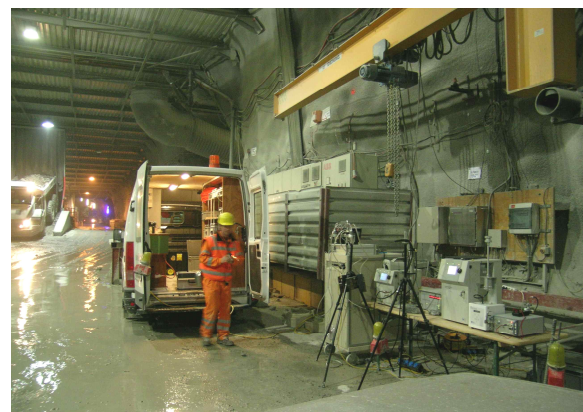
Figure 1: Comparison of different measurement systems in a tunnel construction site.
