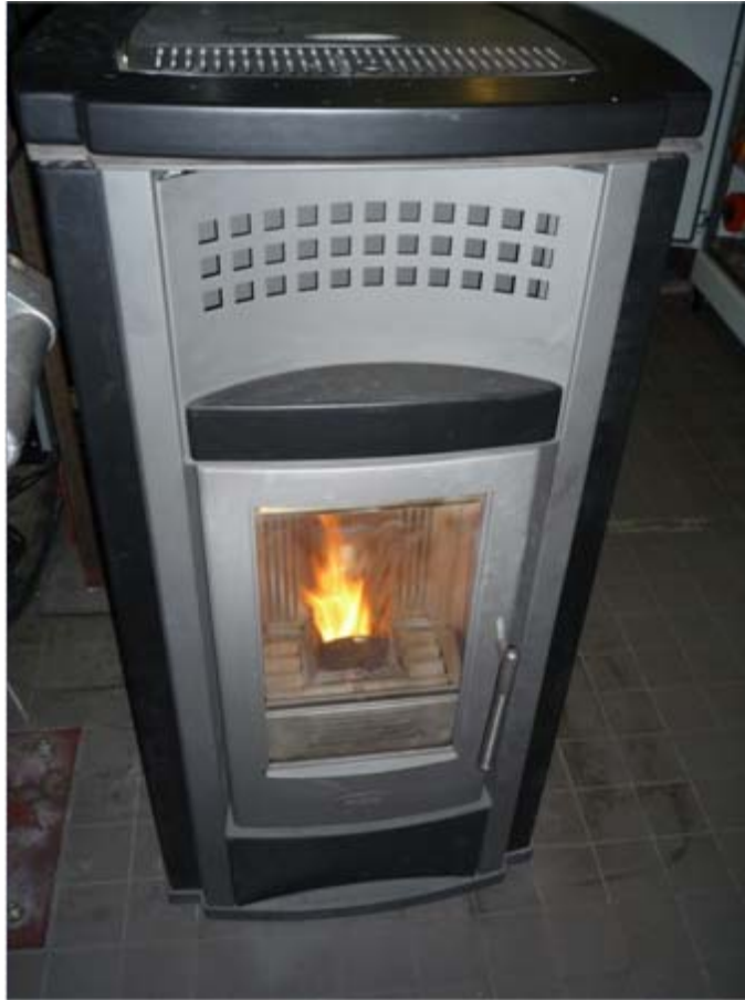
Buderus Blueline Pellet 1 Pellet stove (7.6 kW), manually fed
