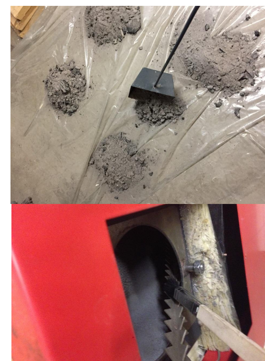
Figure 2: Coarse and filter ash sampling at the logwood boiler
