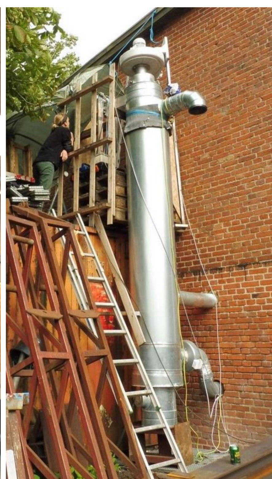
Condensing bag filter system
