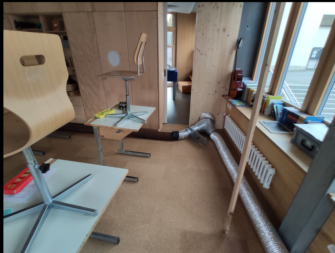
Flow recirculation by fabric-tubes
